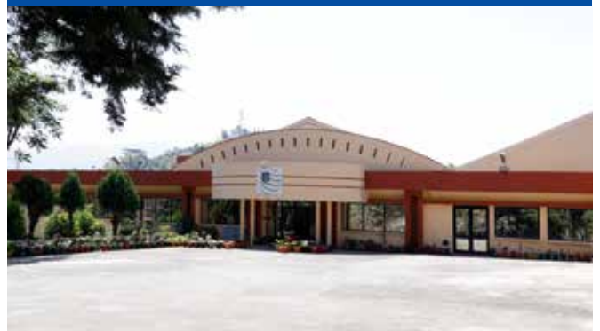
Telecom Equipment Plant, Solan
