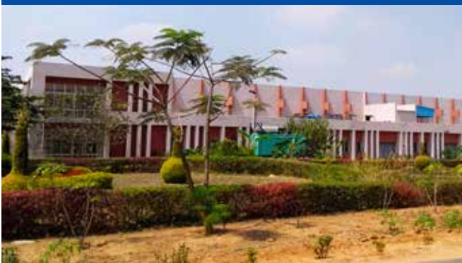
FRP Plant, Hosur#
