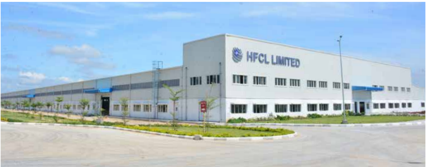
Upcoming Optical Fiber Cable Plant, Hyderabad
